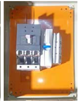
ENCLOSED CIRCUIT BREAKER
